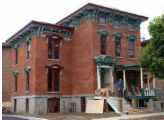
▮ The refurbishing of 3 Steuben Park nears completion.
